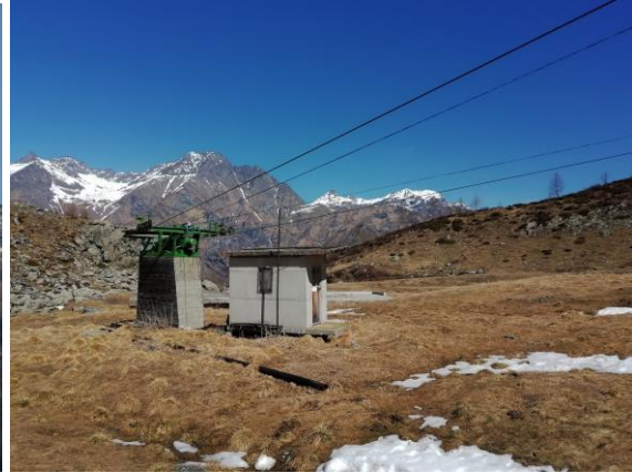
Impianto in disuso a Pian Benot
